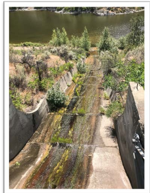
Irrigation Canal Spillway at Mud Lake
