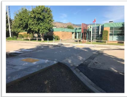
Speed Hump Park Drive
