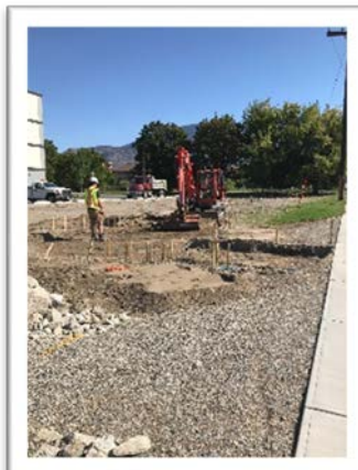
Bridge Park Construction
