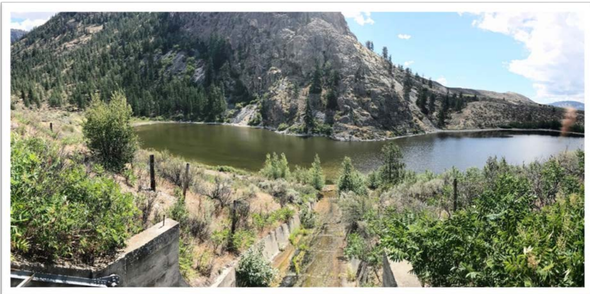
Canal Spillway at Mud Lake
