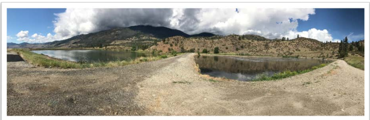
Aeration Cells #2/#3 Topping Lake Treatment Facility
