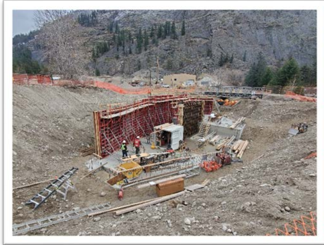
Gallagher Lake Siphon – new pumphouse construction started
