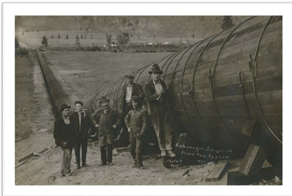
1920 South Okanagan Irrigation Stove Pipe Siphon
