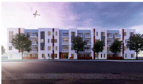
1.0 ■ 1/18 REPORT STREET LOOKING EAST
